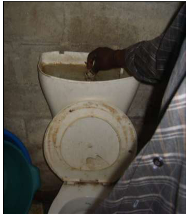
Figure 6. Flushing mechanism on this toilet is broken in a house in Masipumelela. Users flush toilet by manually manipulating the mechanism inside the system. Note that the toilet is dirty.
