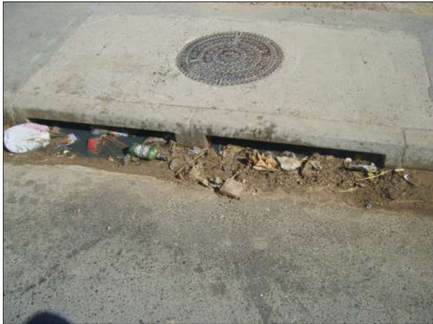
Figure 8. Solid waste blocking the storm water inlet on street causing subsequent flooding during rain storms in Greenfields.
